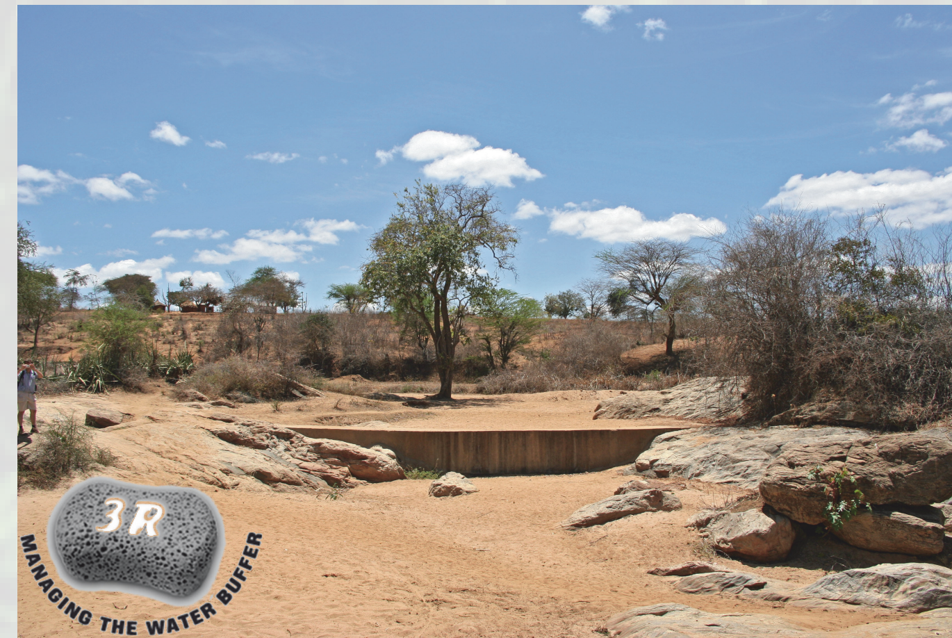
Fig. 1: A typical sand storage dam during the dry season in the Kitui District, Kenya
