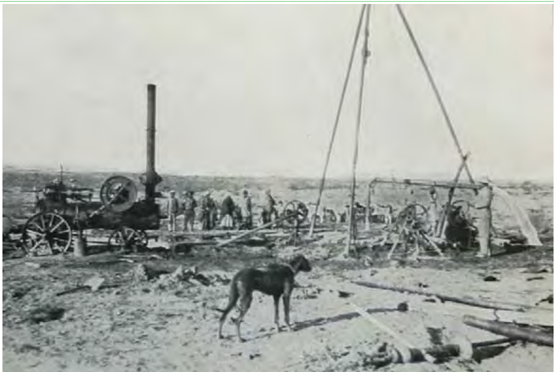
Figure 2.1 | First artesian water was struck in 1912 (110 m 3 /hr free flowing artesian borehole) (Source: National Archives of Namibia)
