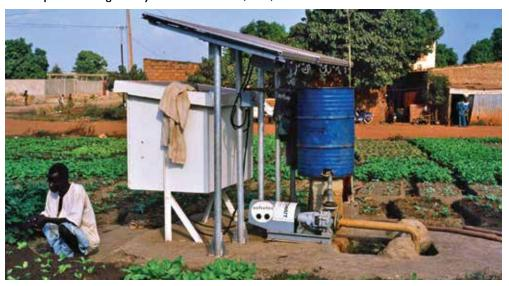
FIGURE 2 A solar-powered irrigation system near Bamako, Mali, 1981
