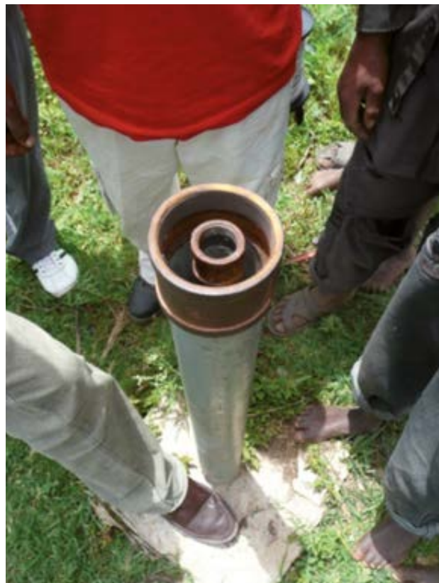
Figure 5.3 Example of a dedicated monitoring well: a 1” or 2” screen pipe with 3 or 4” upper casing that prevent the wells from flooding and allows for a proper screwed cap for protection. 1” observation wells are for water level recordings only (with a water dipper or a diver). 2” observation wells also allow for water sampling with a bailer
